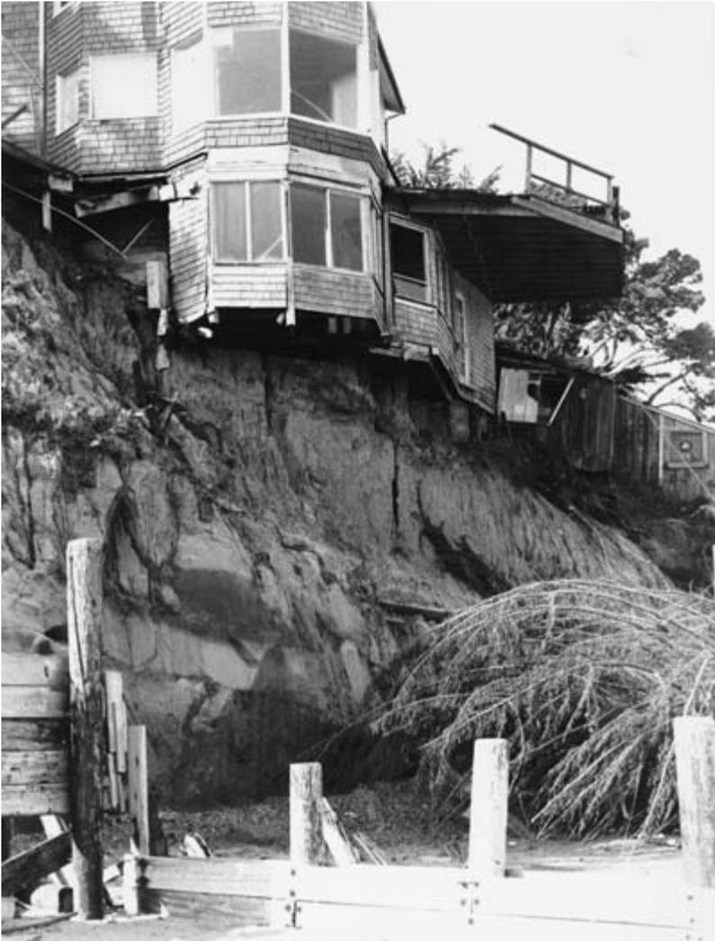
Figure 1.2 House on the side of a bluff at Bolinas undermined by erosion during the 1983 winter. Photo by Gary Griggs and Kiki Patsch.
