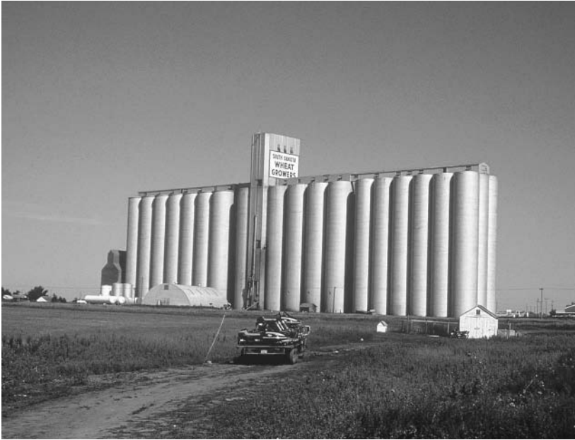
Figure 1.8. Grain elevators near Aberdeen, South Dakota, 1978. The historian William Cronon, in Nature's Metropolis , traces the economic and ecological impacts of the invention of the nineteenth-century wooden grain elevator (far left). The huge, post-1945 concrete additions reflect the expansion and centralization of the world grain market.
