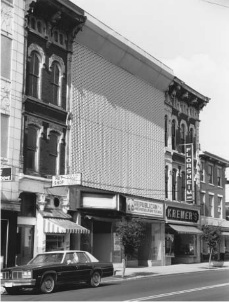
Figure 1.5. Downtown commercial building in Zanesville, Ohio, 1985. Strict architectural preservationists might be most attracted to the design of the original 1870s facade, while a cultural landscape approach might find equal interest in the 1960s aluminum refacing of the center section of the building, and in the first-floor storefronts, each from a different decade.
