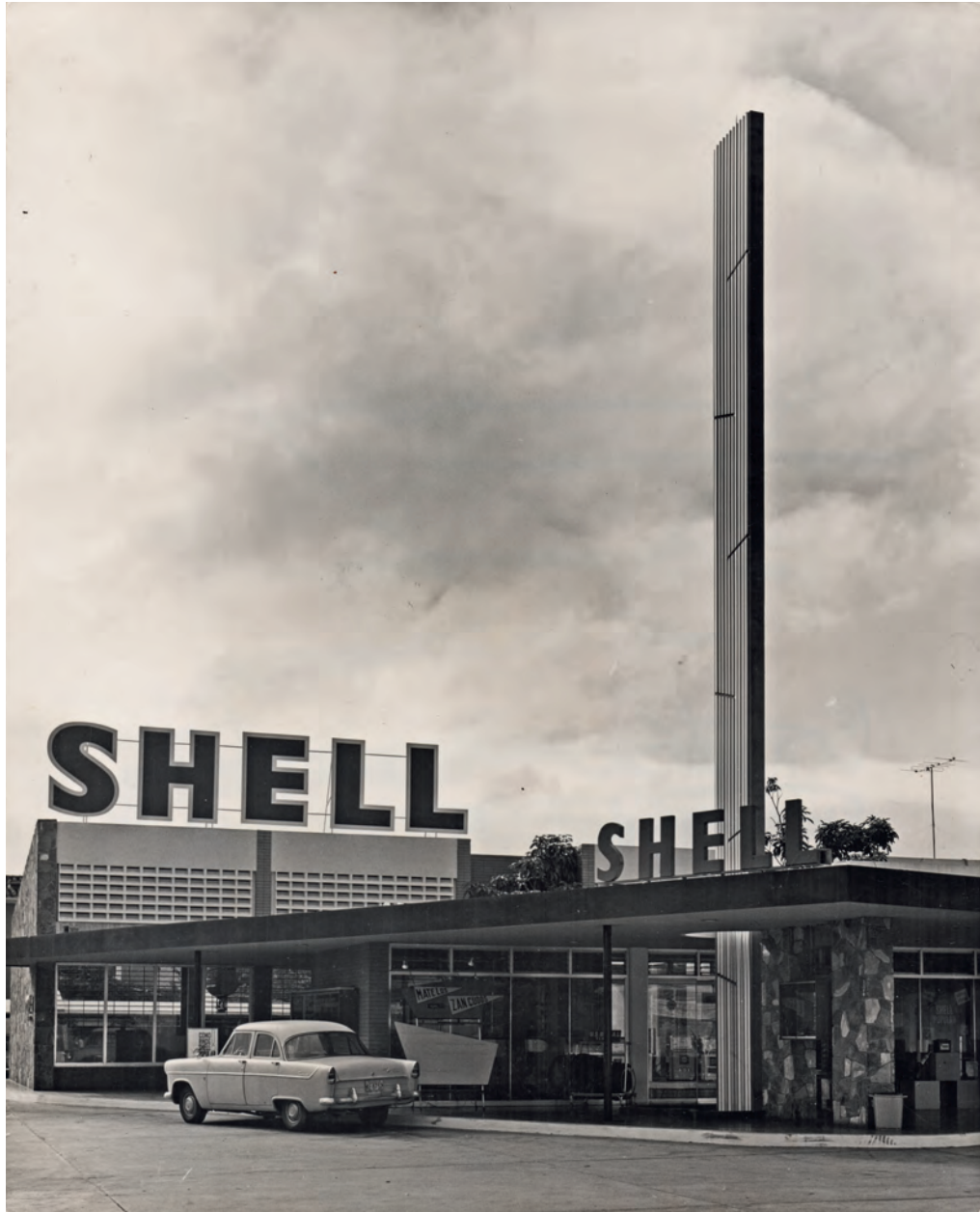
FIGURE I.1. Alejandro Otero, Mástil reflejante (Reflecting Mast), 1954. Corrugated aluminum. Las Mercedes, Caracas. Courtesy of the Otero Pardo Foundation.
