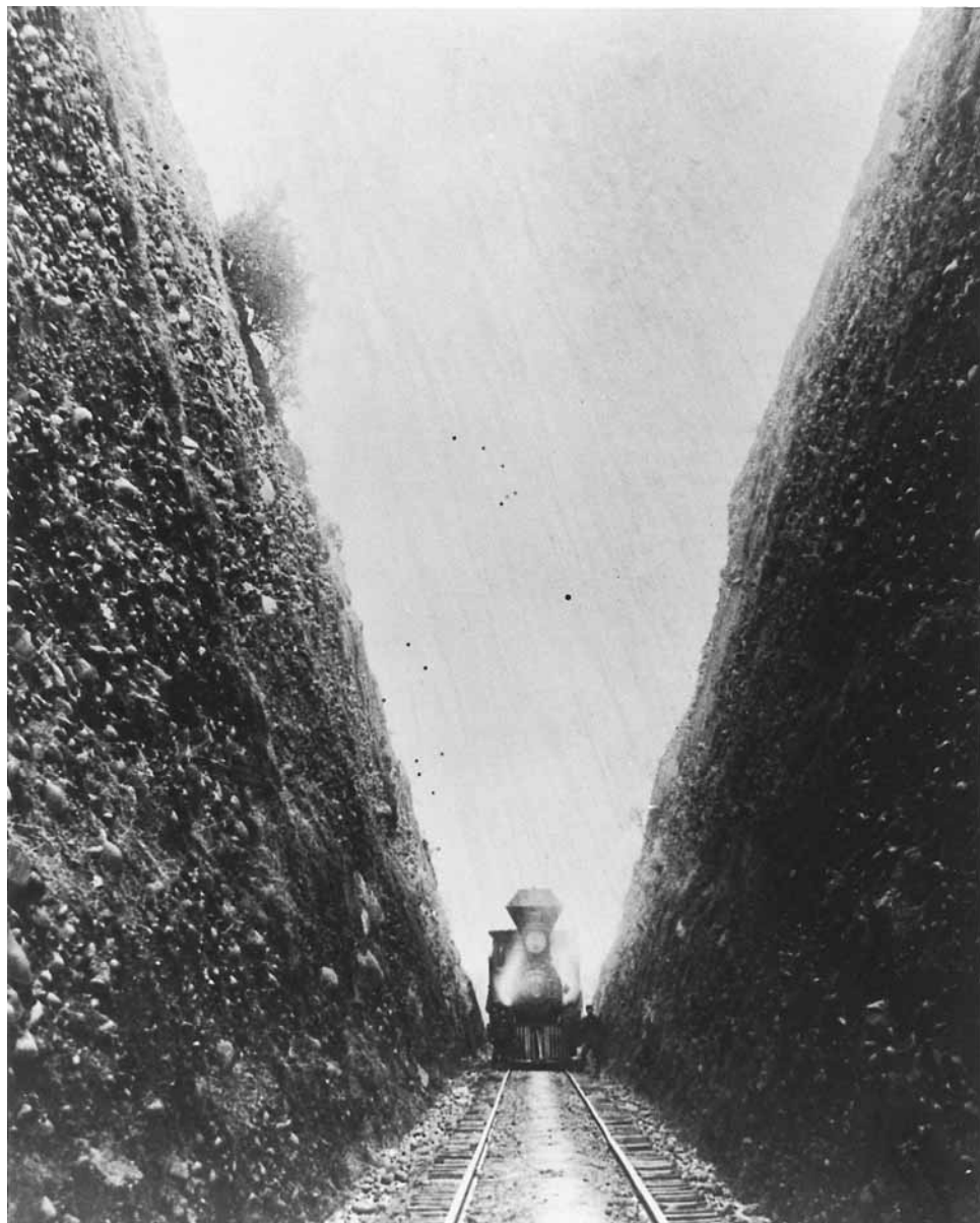
Central Pacific Railroad locomotive in the Bloomer Cut, near Auburn, California, photographed in mid-1860s by the company's photographer, Alfred A. Hart. Building the railroad over the Sierra Nevada was one of the nineteenth century's greatest engineering achievements. Courtesy California State Railroad Museum, Sacramento.
