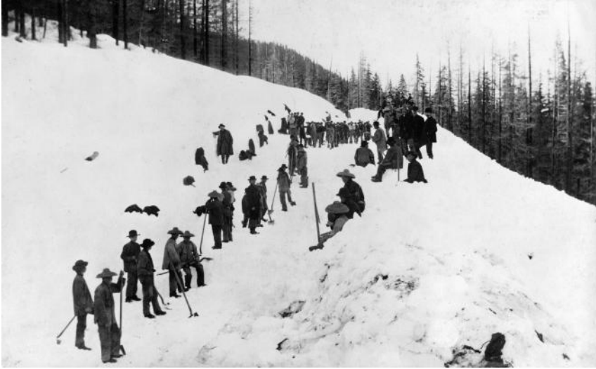
FIGURE 1.4 Chinese workers clearing snow from railroad tracks, 1886. Heavy snowfall sometimes buried tracks so deep that rotary snowplows could not operate. Then it was necessary to employ shovel gangs to clear tracks. University of Washington Libraries, Special Collections, UW552.
